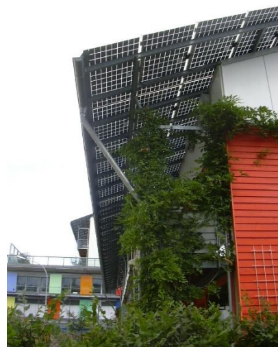
Figure 10. PV roof detail of Solar Siedlung (Müjde Altın archive, August 2006)
