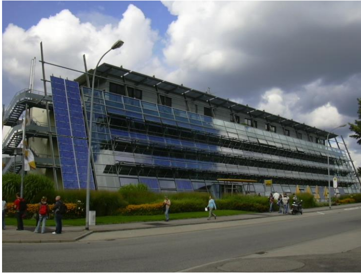
Figure 7. South façade of Solar Fabrik Administration Building (Müjde Altın archive, August 2006)
