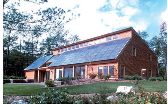
Figure 6. Carlisle House with its roof cladded with PV components (Solar Design Associates, u.d.)
