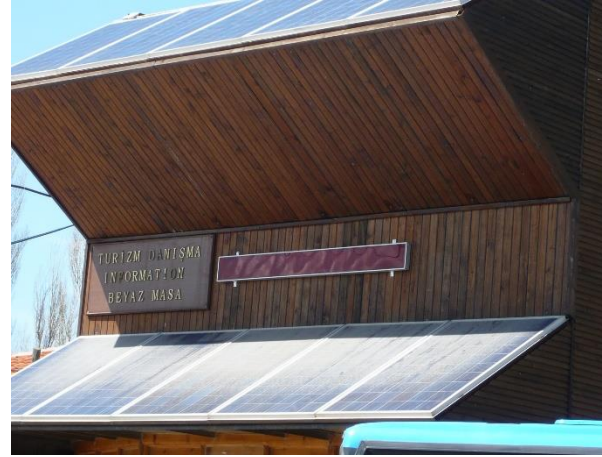
Figure 12. PV detail of Gökçeada Municipality Service Building (Müjde Altın Archive, April 2010)
