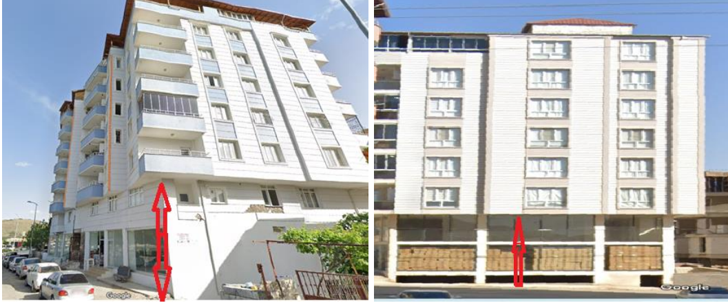
Figure 3. Gaziantep Nurdağı example buildings with soft floors (Google Earth, 2024).
