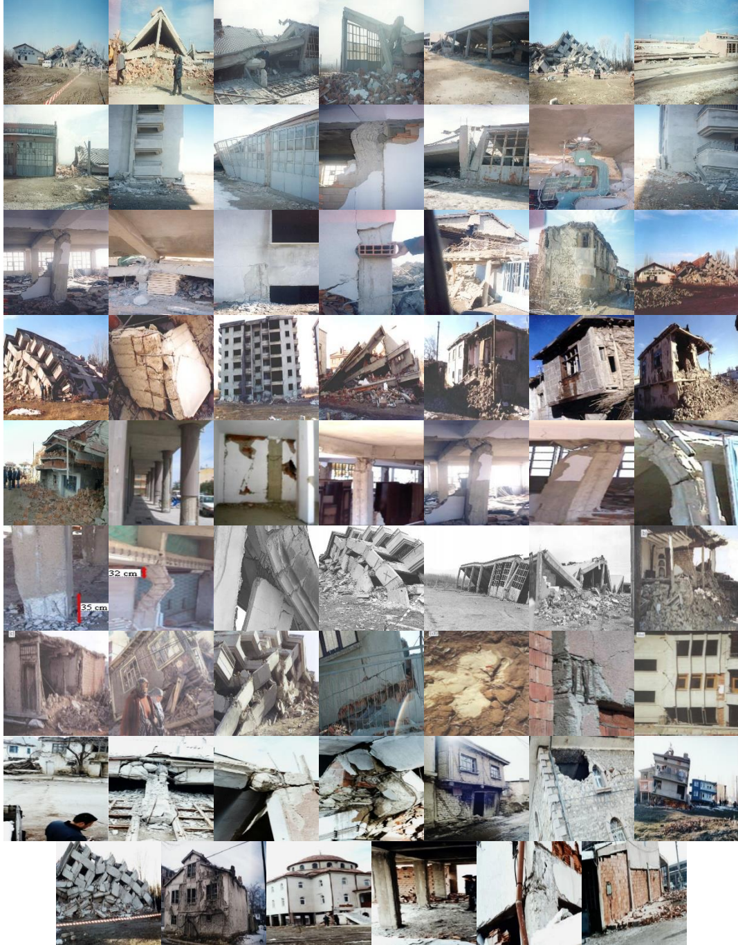
Figure 4. Structural damage photos of the Sultandağı Earthquake
