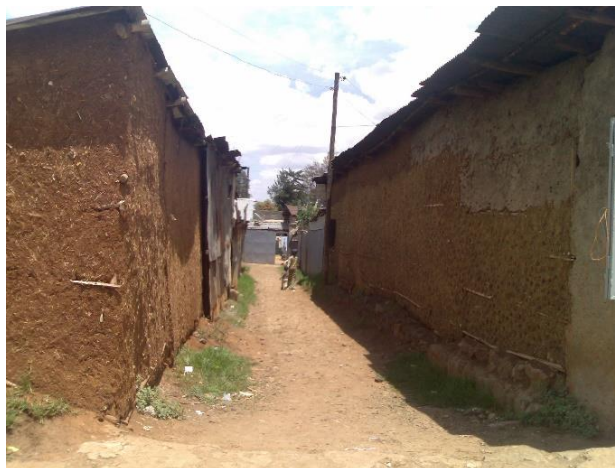
Figure 2. Housing Condition at Slum Areas
