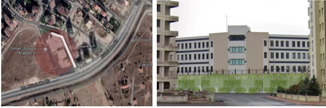
Figure 25. Retaining wall of Osman Ulubaş Mansion Anatolian High School, which is thought to have potential for vertical garden applications.
