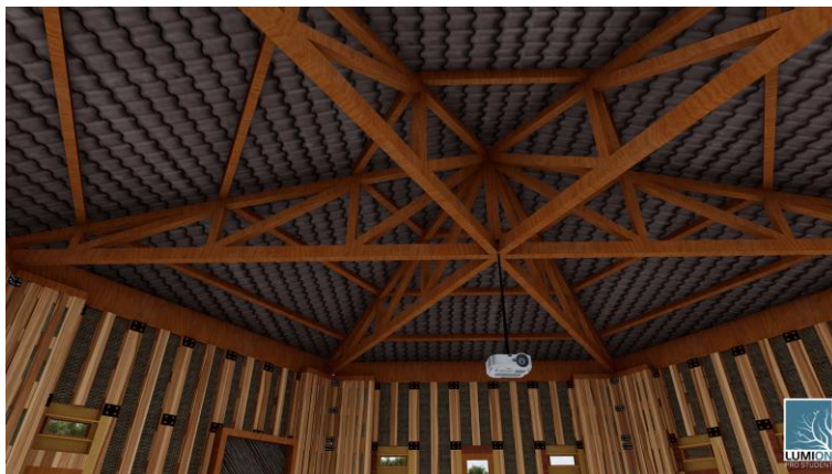
Figure 39. Library building roof detail
